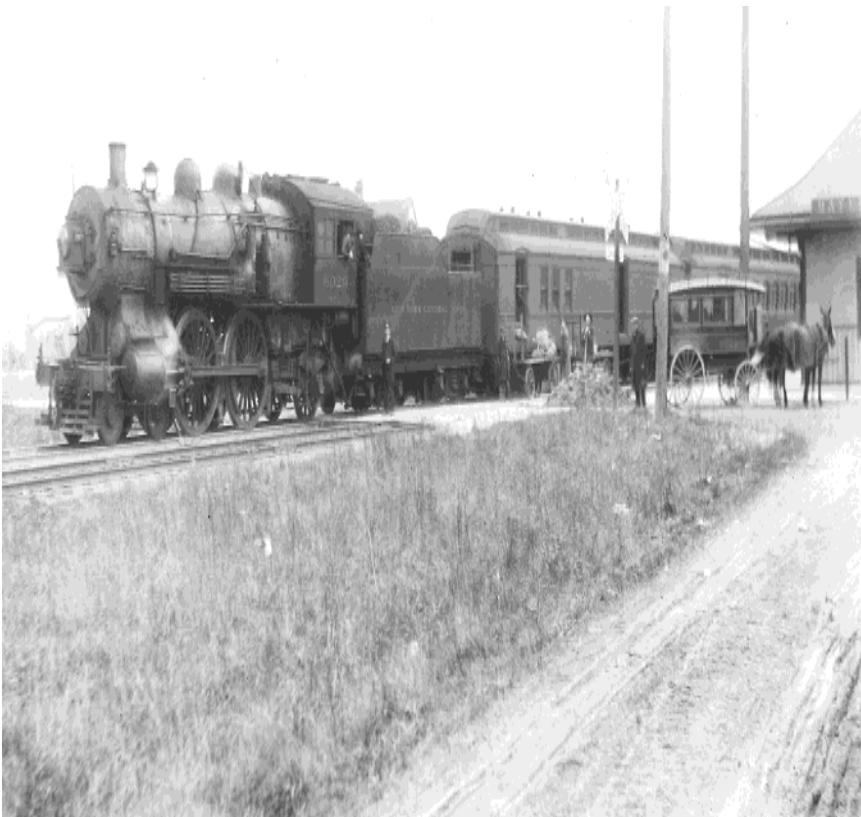
At one point, two trains a day were passing through Batesville including this one arriving from Indianapolis with passengers and freight. This was the New York Central Line, engine number 6929.
